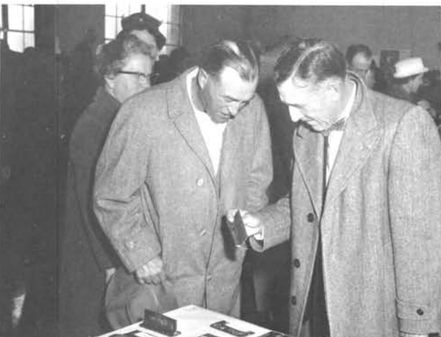
Some fathers are interested in the welding.
