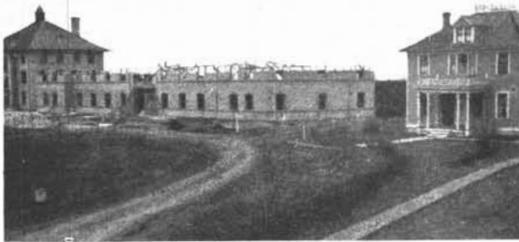
Campus in 1908, Stephens Hall in construction
