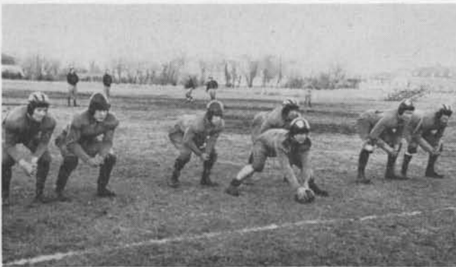
The first string line
