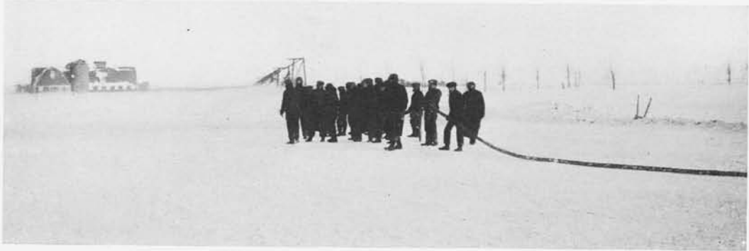
FLOODING THE RINK
